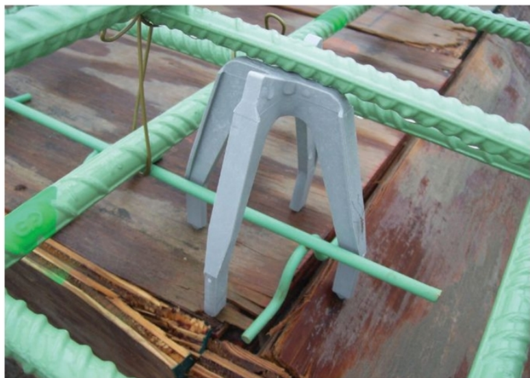
Epoxy-coated reinforcing steel placed on epoxy-coated wire and plastic bar supports. All Photos: EIG.
